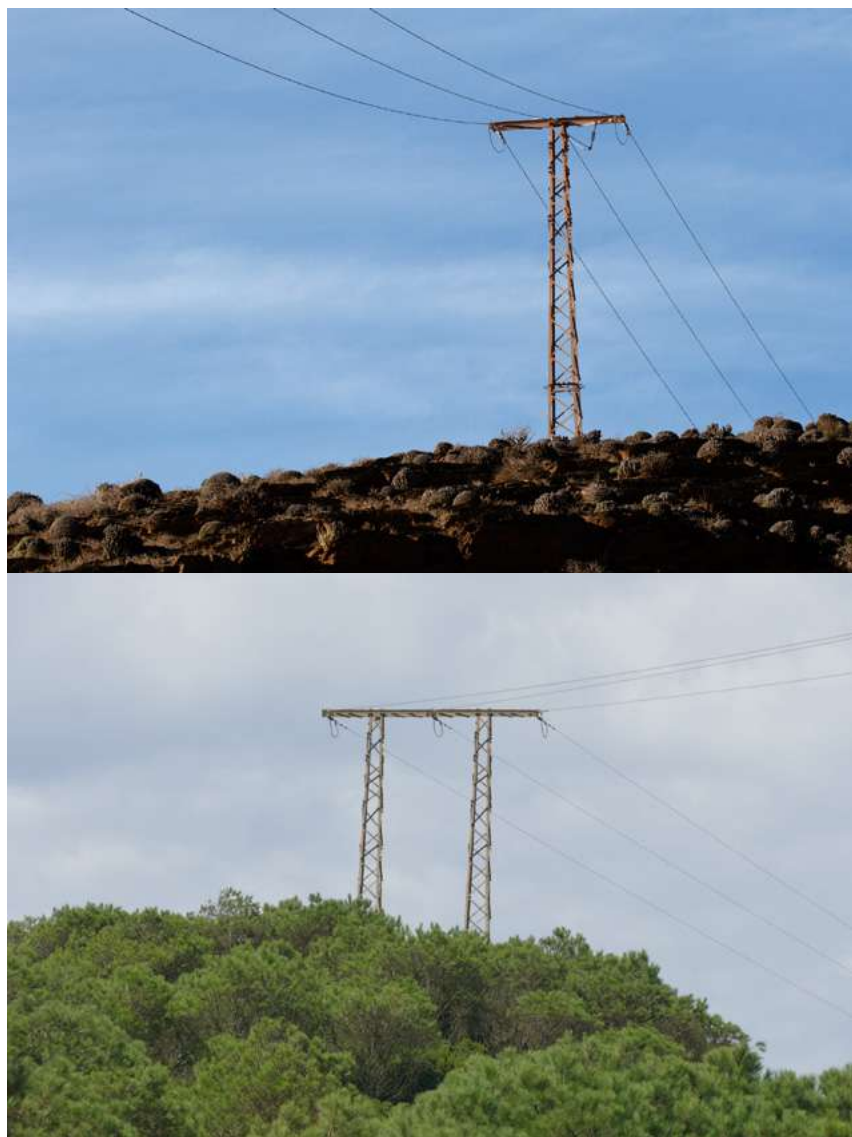
Figures 44 and 45. Anchor pylons can be divided into strainer pylons (above), built in straight lines, and dead-end towers (below), at the start and end of a line and at branch points. ©Daniel Burón (above) and Justo Martín (below)
