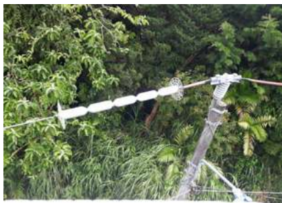
Figure B9. Arrangement of spikeless rotating barriers on conductors.
