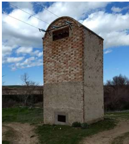
Figures 38 and 39. Examples of distribution substations located inside their own buildings. The (bare) medium-voltage line enters the building and the (sheathed) low-voltage lines carry electricity to the end consumers. © GREFA electric power line team
