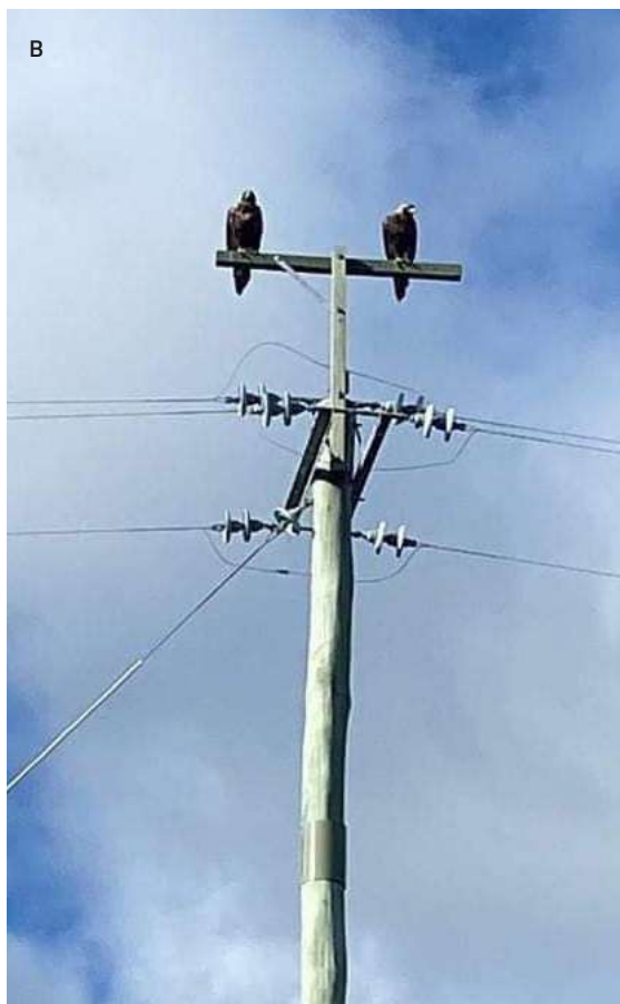
Figure 205. A: Wedge-tailed eagle ( Aquila audax ) on power pole. B: Adult and juvenile wedge-tailed eagles perched on a pole-top perch added to keep raptors from pole-top wires, near Ross in central Tasmania, July 2020. ©Peter Thorpe
