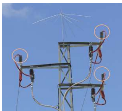
Figure 128. Dead-end tower with bare connections to surge arresters on conductors. © Justo Martín
