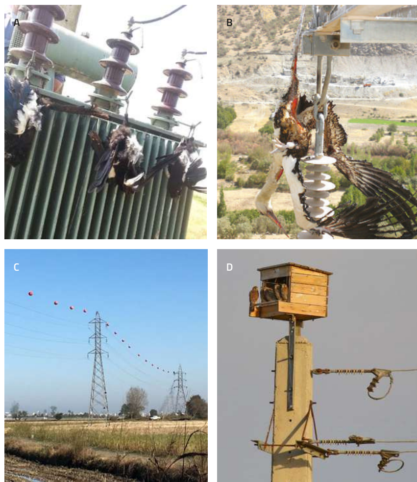
Figure 197. A and B: Bird mortality due to electrocution. A: Electrocution of three Eurasian magpies ( Pica pica ) on arcing horns of a 20 kV pole-mounted transformer. © IBPLC. B: Electrocution of a white stork ( Ciconia ciconia ) on a 63 kV power pole. © Mohammad Sadegh Arshadi. C and D: Retrofitted power lines in Iran. C: Retrofitted transmission line with red bird balls, Mazandaran province, Iran. © Mohammadali Yektanik. D: A wooden nest box installed on a distribution power pole, Markazi province, Iran. © Mahmood Kolnegari
