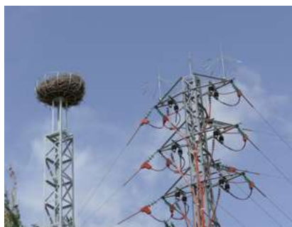
Figures 117 to 120. (From left to right, top to bottom). Further examples of anti-perching deterrents. Figure 117. Raised perch on top of the pylon combined with anti-perching deterrent; white stork. © Justo Martín. Figure 118. Anti-perching spikes. © James Dwyer. Figure 119. Raised platform for nesting; white stork nest. © Justo Martín. Figure 120. Combination of perching deterrents with an alternative artificial nest nearby. © Justo Martín
