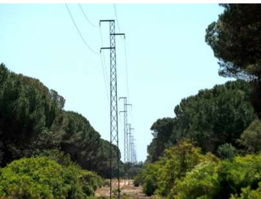
Figure 67. In wooded areas, the risk of collision is higher when conductors pass just above the treetops. ©Íñigo Fajardo
