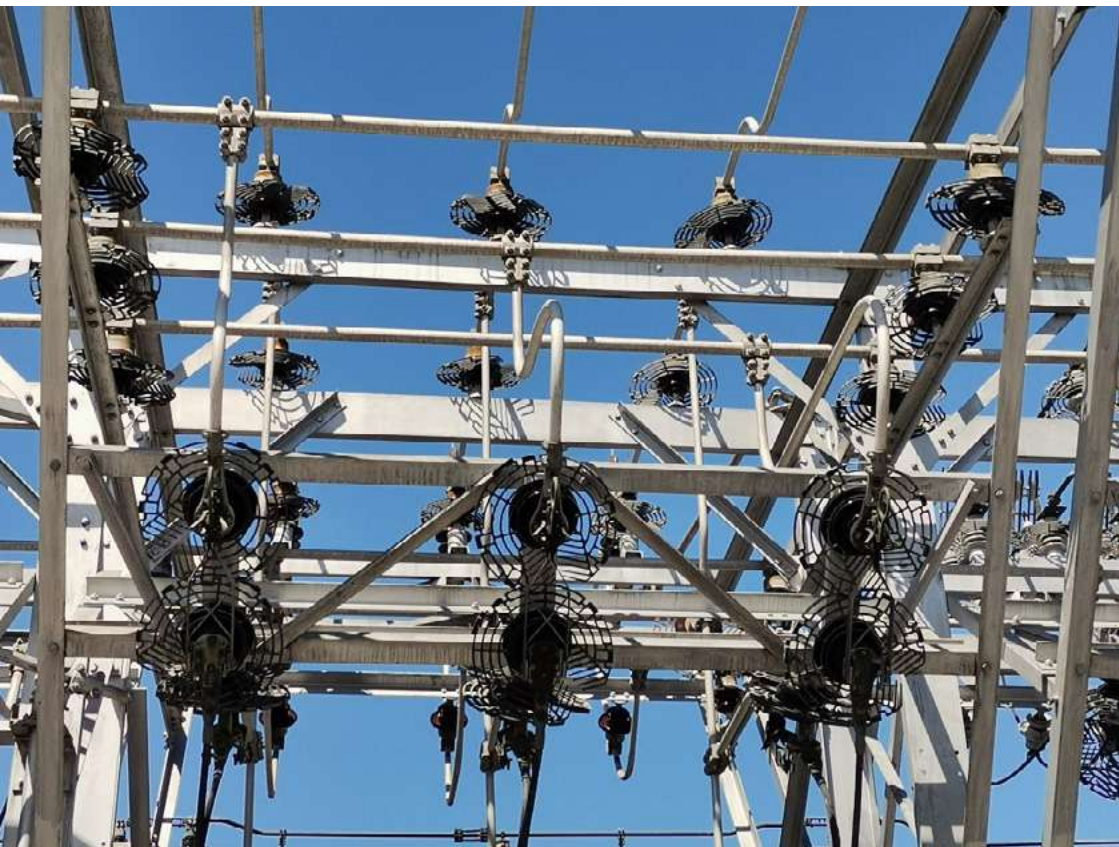
Figure B12. Electrostatic devices fitted to the porcelain fuse cut-out insulators in a substation: design and correct installation. © Ezequiel Herrera/CNFL
