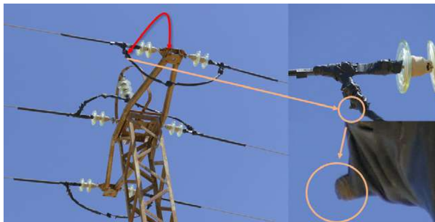
Figure 131. Old, deteriorated insulation in which metal parts (circled) are currently uncovered, posing a risk of electrocution if a bird perches on the crossarm (red arrows). © Justo Martín
