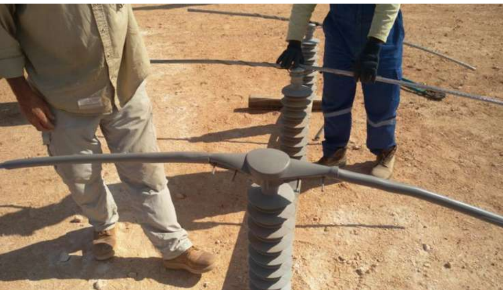
Figure 108. Coverings consisting of preformed parts are the type of insulation most commonly used. Silicone is one of the materials used to make these pieces, since it provides high strength and durability. © Imad Kanouni
