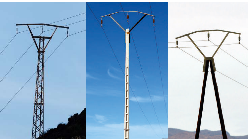
Figures 27, 28 and 29. Supports are built of metal (left), concrete (centre) or wood (right). ©Daniel Burón
