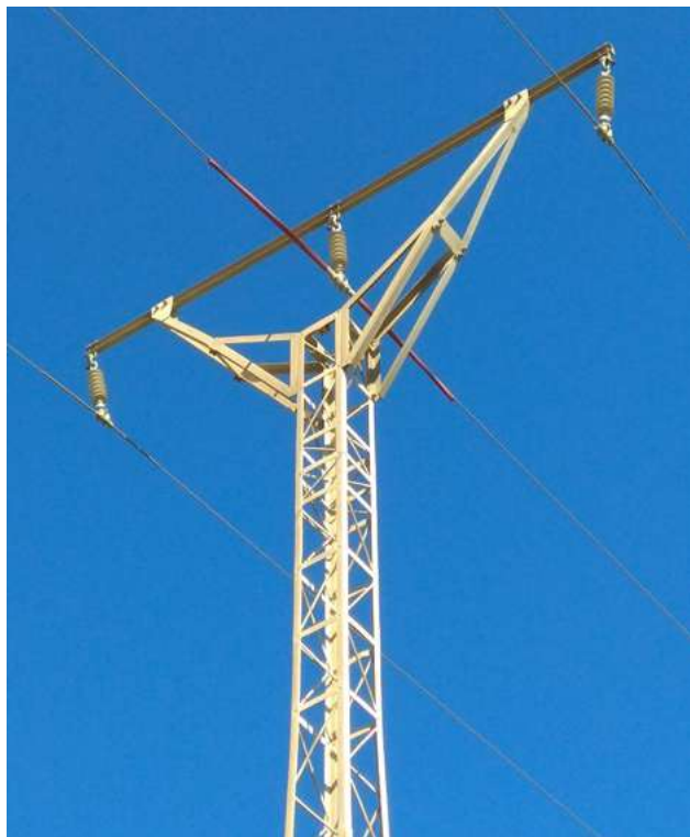
Figure 130. Pylon with vault crossarm configuration on which the central conductor is insulated in order to avoid the electrocution of birds that perch on the base. The risk of defecation is also avoided in this position, but not at the ends of the crossarm, where the layout allows birds to perch. © GREFA Power Lines Team
