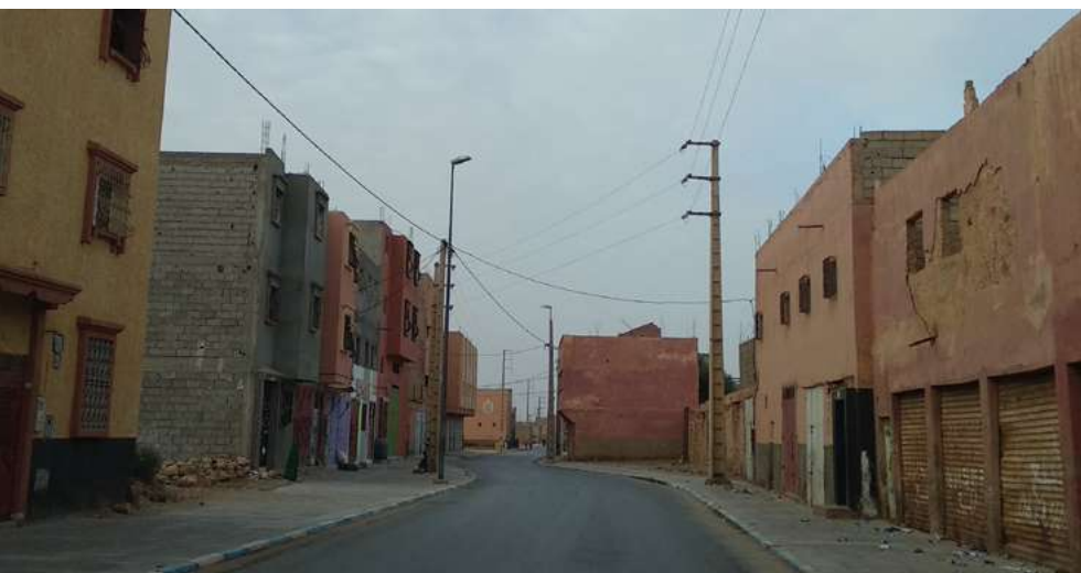
Figure 25. On the left, low-voltage line, with sheathed, twisted conductors; on the right, medium-voltage line with three bare phase conductors. © Justo Martín
