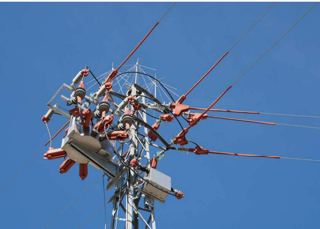
Figure 12. There is the scientific, engineering and industrial capacity to implement effective prevention and mitigation measures. Pylon retrofitted with different types of insulation devices. © Justo Martín
