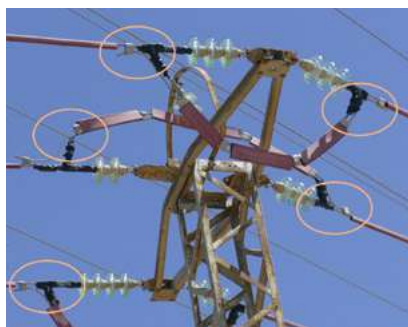
Figure 124. Installation of insulating devices in which numerous metal parts remain uncovered close to the area where birds perch. © Justo Martín
