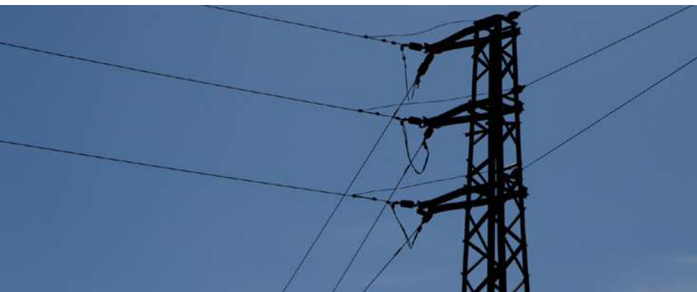
Figure 46. Derivation pylon with a single crossarm assembly and without cut-out fuses or disconnectors. © Daniel Burón
