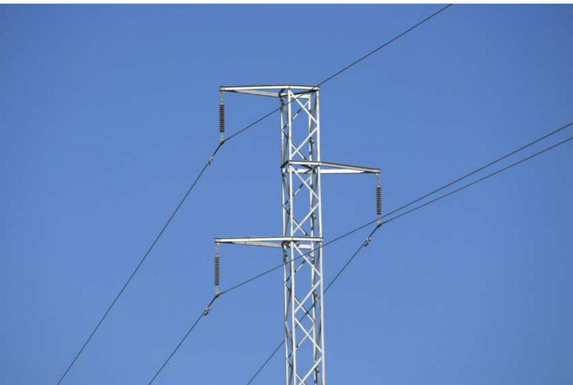
Figure 105. The use of a bird-safe design is the best measure to minimise the risk of electrocution. Crossbar with suspended insulators in alternating arrangement, with safety distances between critical points. ©Justo Martín
