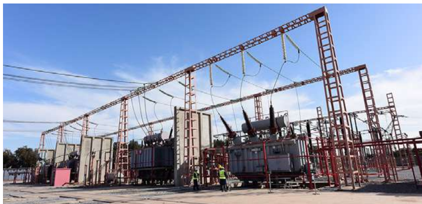
Figure 21. In substations, the electricity from transmission lines is stepped down in voltage and then transferred to distribution lines. Substation in Morocco. © ONEE
