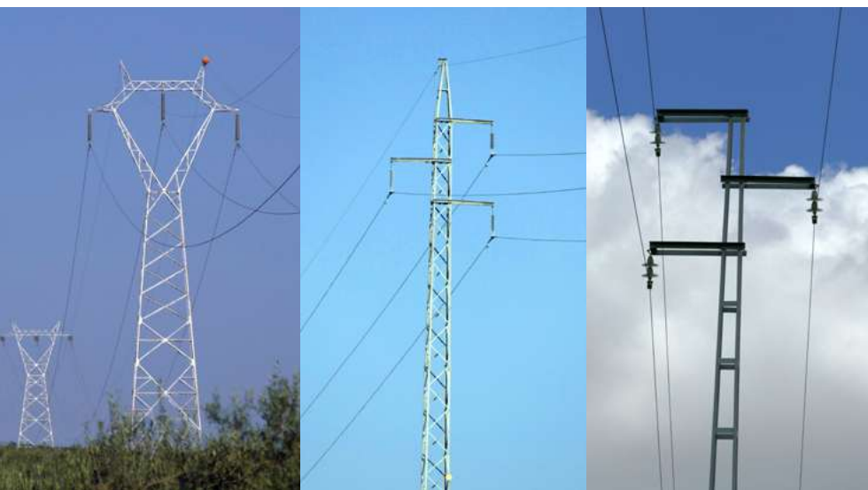
Figures 41, 42 and 43. Left: Pylons carrying a 220 kV transmission line. Centre: Pylon carrying a 66 kV high-voltage distribution line. Right: Pole with a 15 kV medium-voltage distribution line. © Justo Martín
