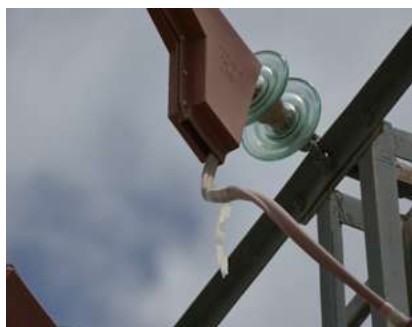
Figure 123. If poor-quality materials are used, defects can quickly appear. Fixation system becoming detached from the conductor just months after it was installed. © Justo Martín
