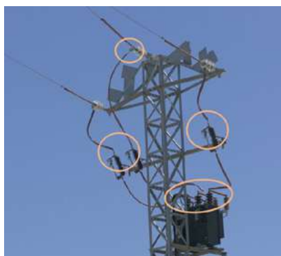
Figure 129. Insulated termination pylon with a transformer, in which the connections between the transformer and the fuses are bare. The upper parts are not correctly fitted, leaving the metal elements uncovered. © Justo Martín
