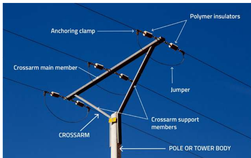
Figure 31. Parts of a support (anchor pole with a crossarm in a vault-type configuration and jumpers under the insulators). ©Daniel Burón
