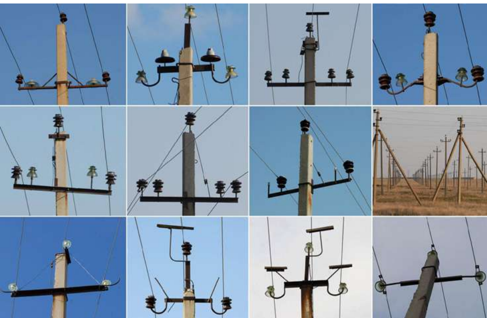
Figure 201. The most common types of 6–10 kV power lines that are dangerous for birds in Russia. Source: Collage from the Russian Raptor Research and Conservation Network (RRRCN) website ( http://rrrcn.ru/ru/electrocutions/pop1 )
