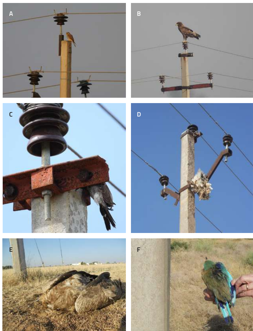
Figure 195. A–D: Three-phase tangent units without any added equipment are the most common configuration. They have the potential to kill both large and small birds (E and F). A: Common kestrel ( Falco tinnunculus ) and B: Indian spotted eagle ( Clanga hastata ) perched on 33 and 11 kV power poles respectively. C: Red-vented bulbul ( Pycnonotus cafer ), D: Indian eagle owl ( Bubo bengalensis ), E: Tawny eagle ( Aquila rapax ) and F: Indian roller ( Coracias benghalensis ) killed on 11 kV power poles. © Pranay Juvvadi
