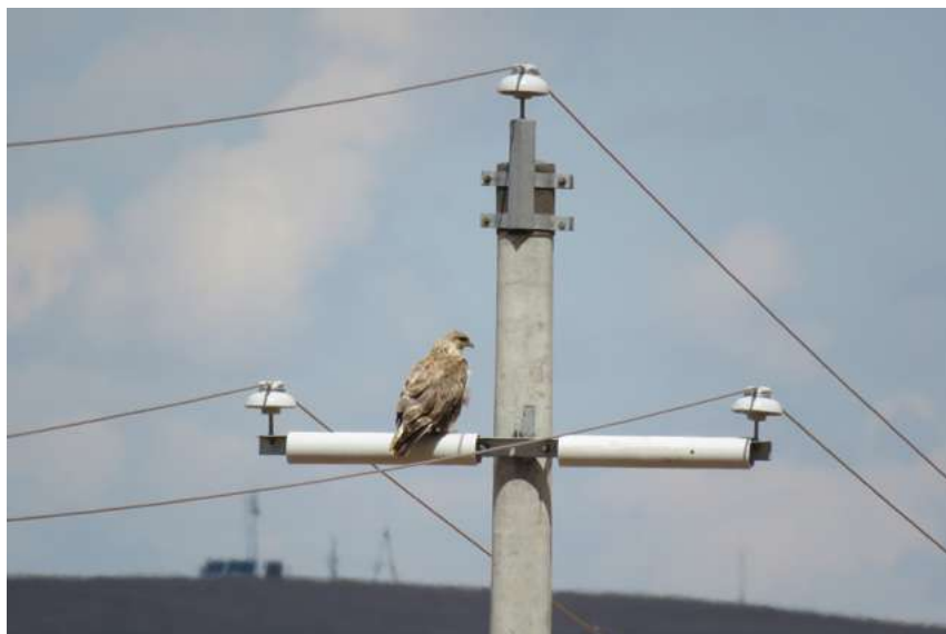
Figure 112. In some configurations, fitting rigid plastic sheaths on the crossarm is a good way of making them safe. Upland buzzard ( Buteo hemilasius ). © Mohamed bin Zayed Raptor Conservation Fund project – Mongolia
