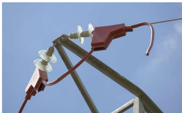
Figure 126. Insulation sheath that has become detached at the end due to poor fitting. © Justo Martín
