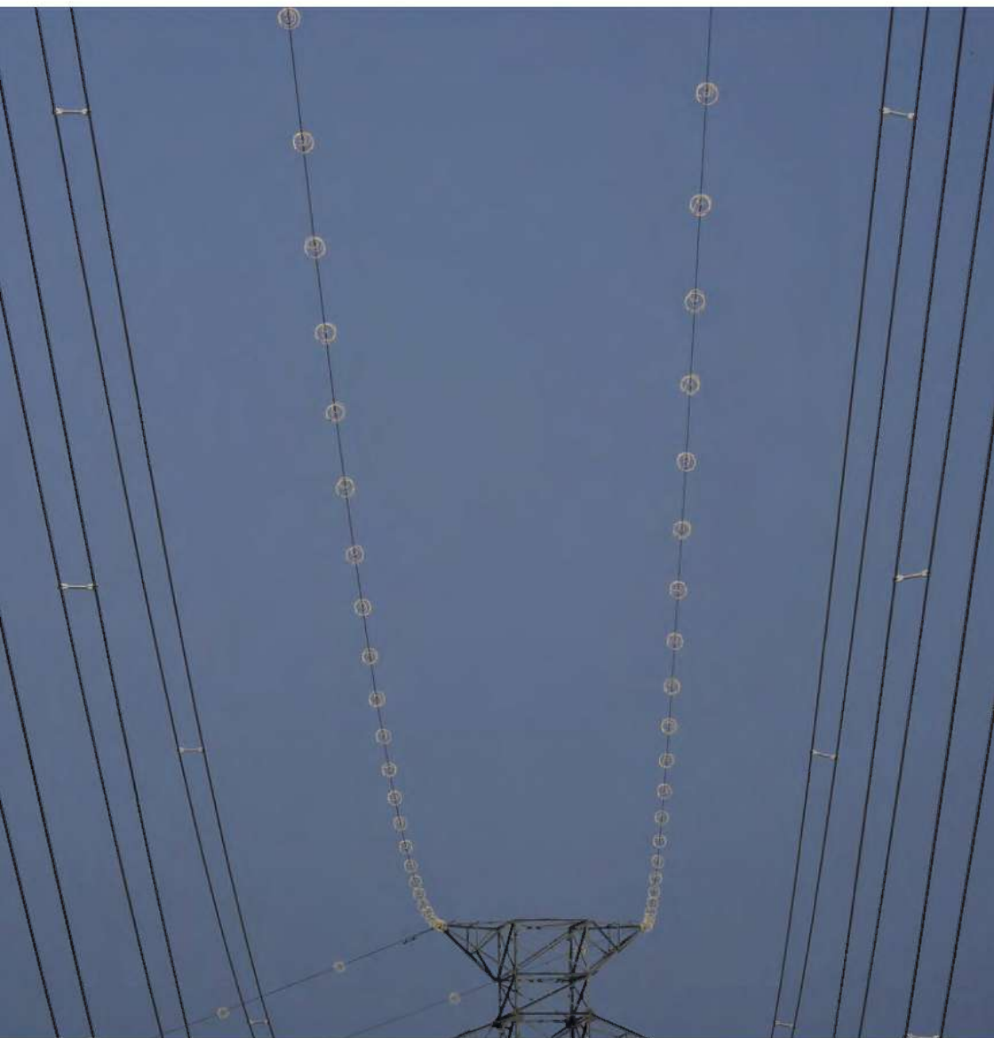
Figure 76. Line markers installed in an alternating pattern on two overhead ground wires of a transmission line. © Justo Martín
