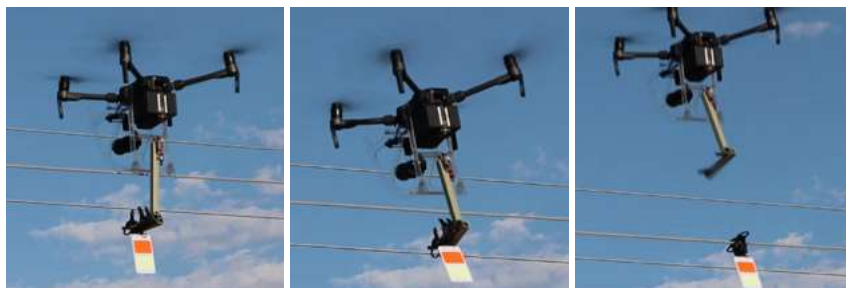
Figures 80, 81 and 82. Installation of flight diverters by drone. ©James F. Dwyer and Richard E. Harness
