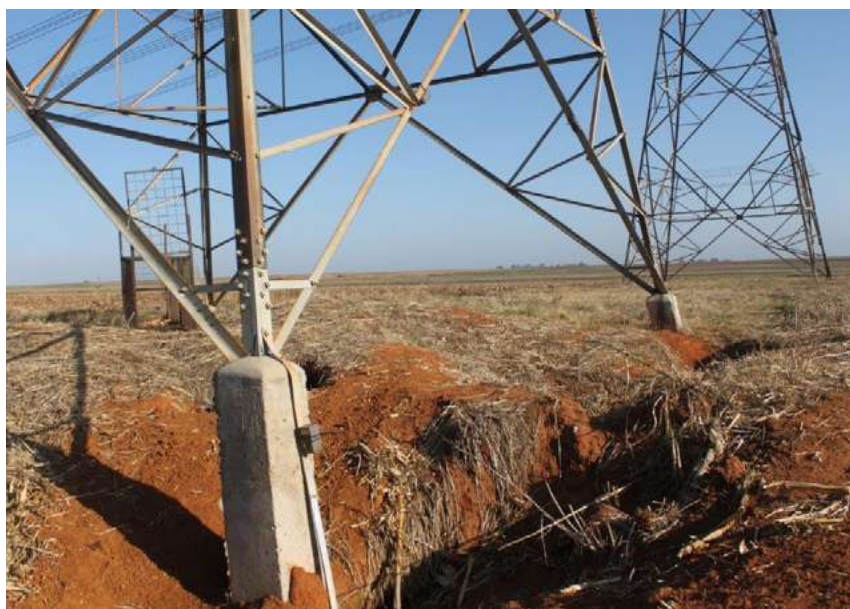
Figures 60 and 61. Damage around the steel lattice structures of a transmission power line caused by African porcupines. © Eskom/Endangered Wildlife Trust Strategic Partnership.
