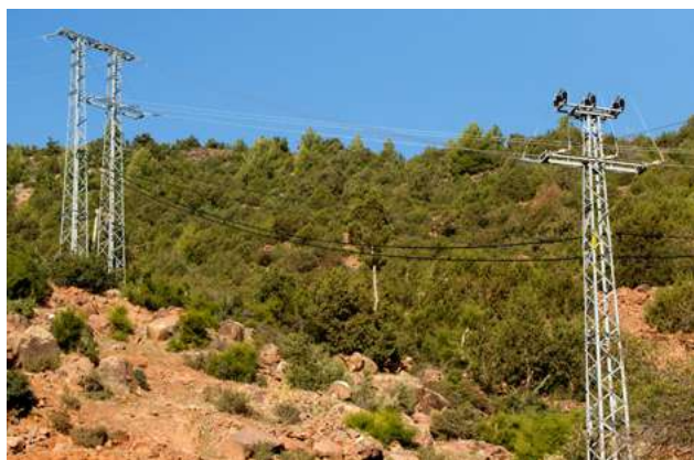
Figure 100. Electrocutions are concentrated on supports with a dangerous configuration and/or where the topography and habitat favour their use by birds or by other animals, and where food is plentiful. Power line with very dangerous pylons, raised above the surrounding vegetation. © Daniel Burón
